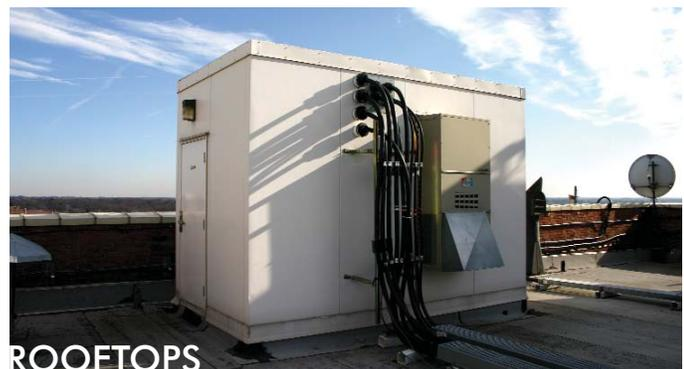
Unassembled or pre-assembled, Enviro Building's rooftop shelters will save you money. The lightweight construction reduces on-site structure support and in return, decreases costs of site preparation. The unassembled modular shelters can also be taken up via elevator and assembled on the rooftop, eliminating the need for a crane.
