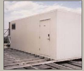
Enviro Buildings' modular product line allows the customer to assemble their own communication shelter on-site for unique locations. Each panel is equipped with a cam-action locking system which enables the assembly of a complete shelter in less than four hours.
