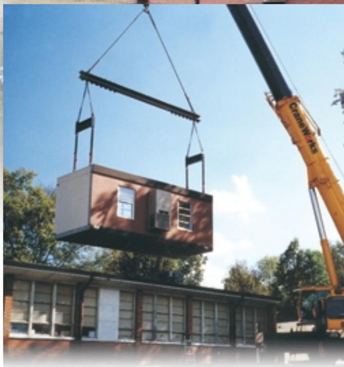
ROHN Concrete Building Systems can provide a cost-effective alternative to traditional site-built structures. They surpass site-built construction in strength, durability, and thermal efficiency. ROHN's Concrete Buildings offer long-term value and flexibility since they can be disassembled and relocated if necessary.
